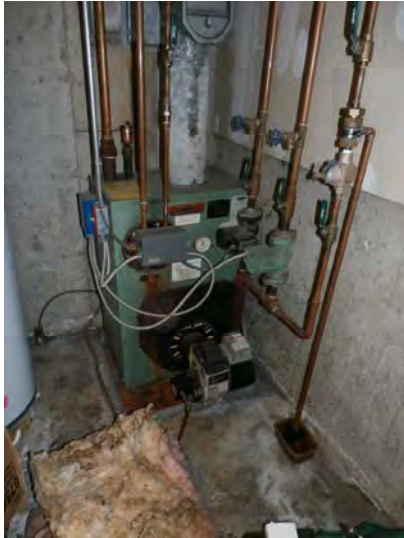
Typical oil-fired hydronic boilers
